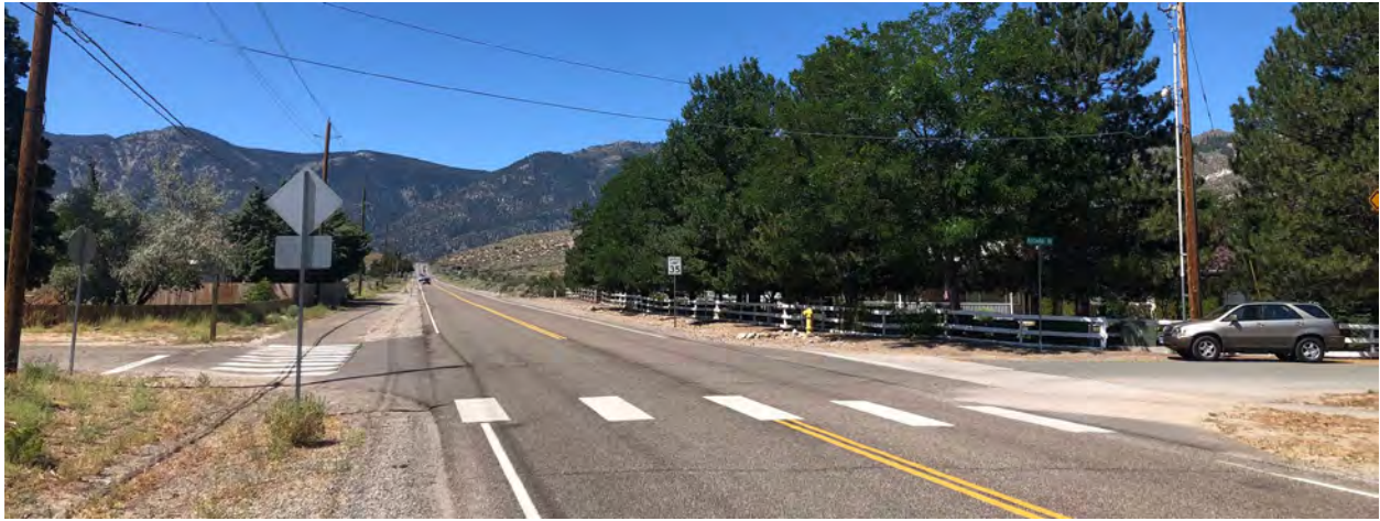
Existing conditions at Jacks Valley Road and Arcadia Drive
